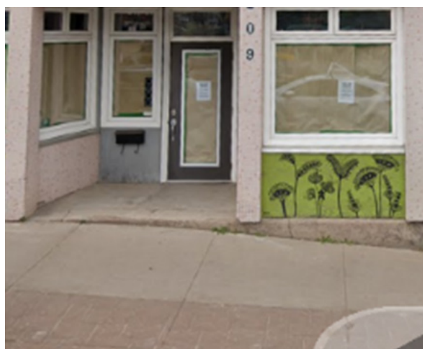
Figure 17. A business entrance in New Glasgow, NS, with an irregular transition from the sidewalk. (Source: Google Streetview)
