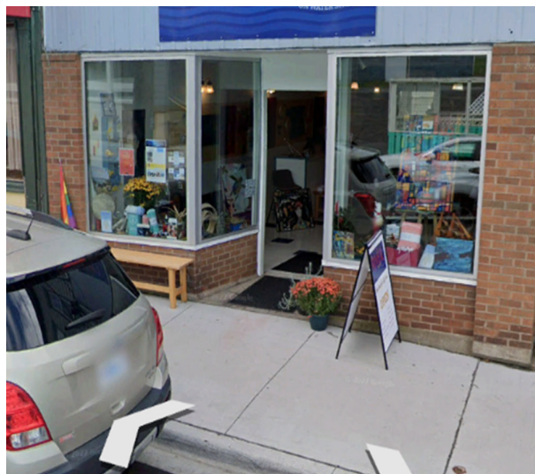
Figure 16. A storefront with a level entrance in Pictou, NS. (Source: Google Streetview)
